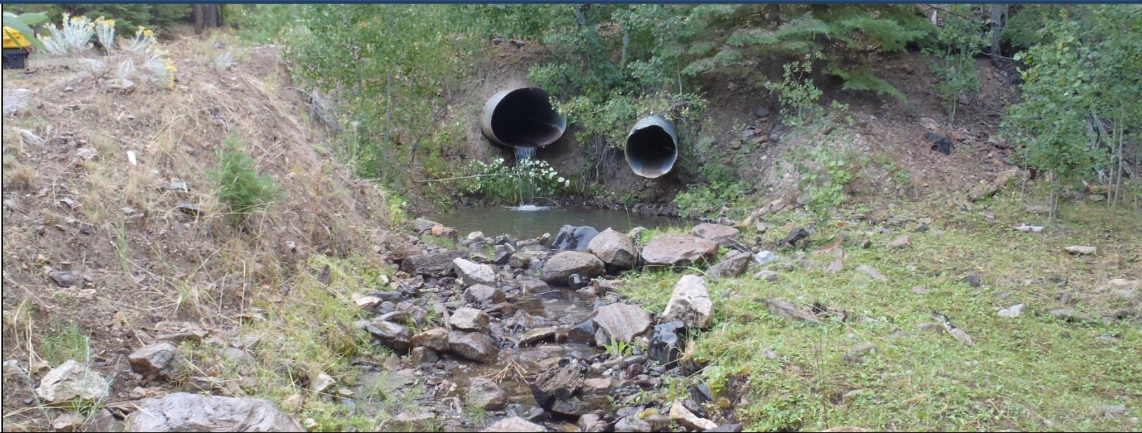
A view upstream to the Howard Creek culverts.
